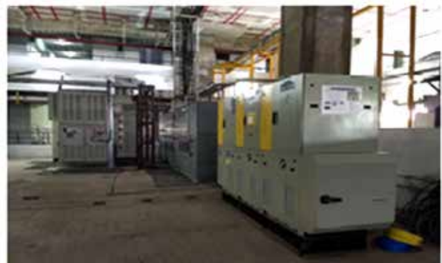
330 kW Power Conditioning Units (PCUs) installed at CDAC-Pune
