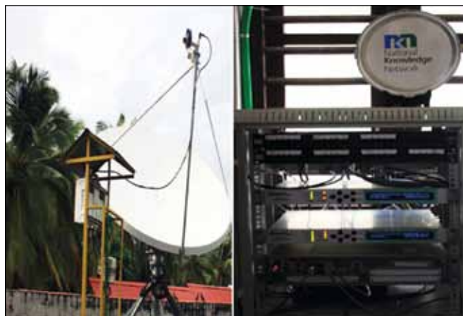
Figure: High Capacity SCPC VSAT at Kavaratti, the U.T. of Lakshadweep Island for NKN
