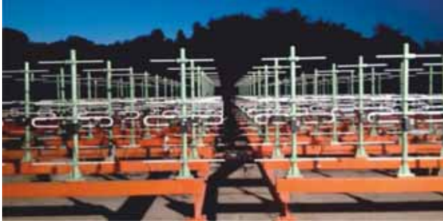
ST Radar Installation work at site is in progress
